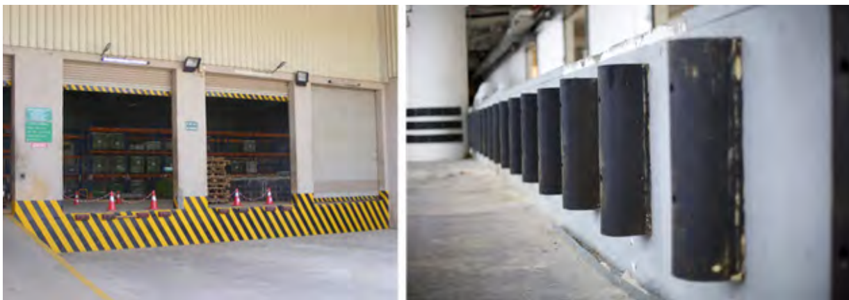
Fig 2.7.7: Loading/ Unloading bay
